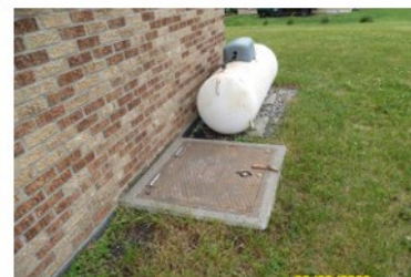
Existing Hatch and Propane Tank
