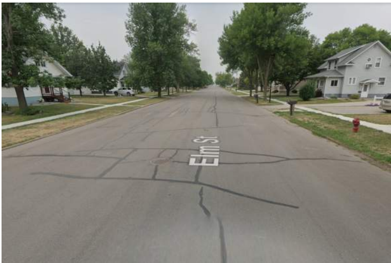
Elm Street looking west (2021)
