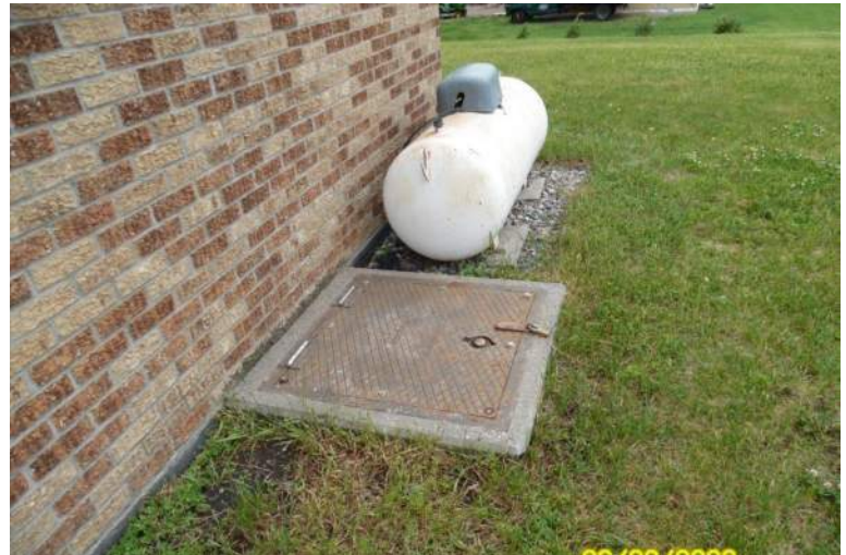
Existing Hatch and Propane Tank
